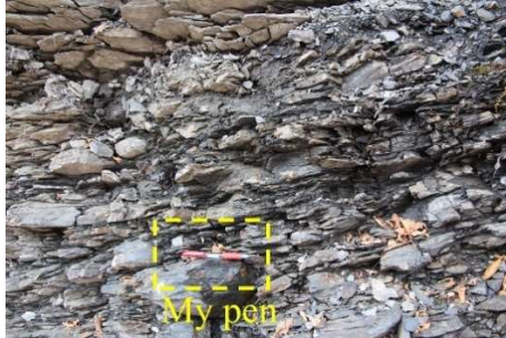
Fig. 12. Fractured rock of Ohya landslide site.
