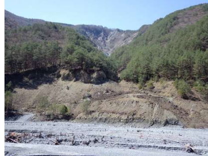
Fig. 26. Tobigasu slope failure along MTL
