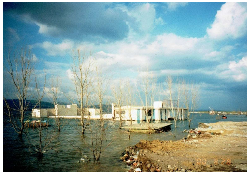
Fig. 36. Subsidence of the coast line of the Izmit Bay.
