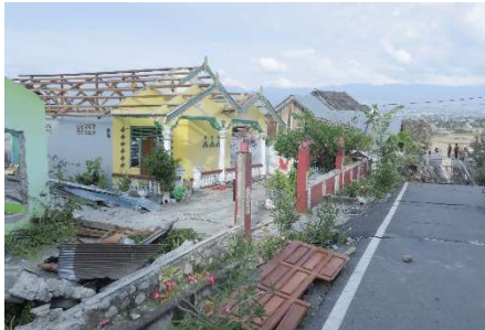
Fig. 40. Lack of irrigation channel above the headscarp of Balaroa landslide.
